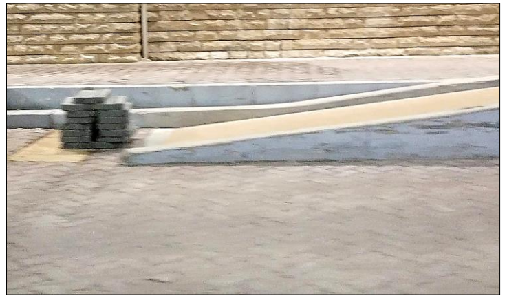
These two steps in front of a grocery store run the entire block. At the far end is a small ramp (no handrails) and it is blocked by a stack of bricks.
